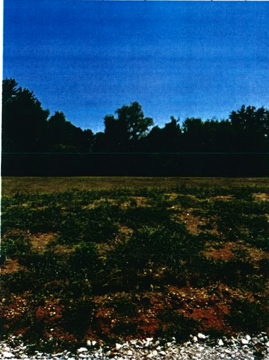
View of South Side of Property from Storage Area – Note Heavy Landscape Screen
